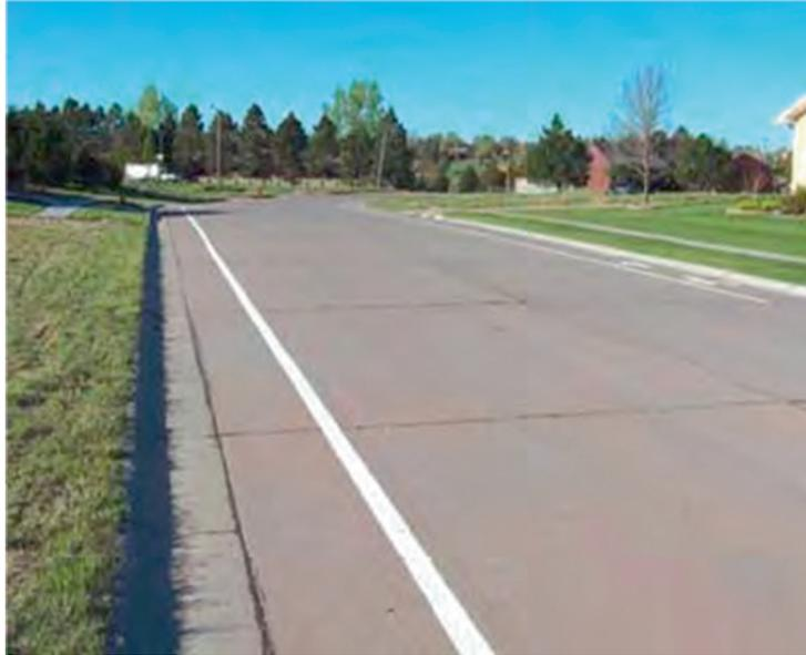
*Figure 1* — RCC pavement on a local road
